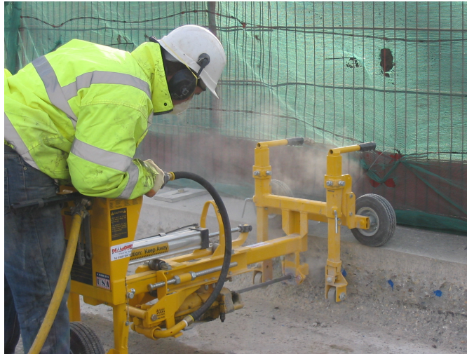
Automated Rock Drilling Alleviates Hand and Arm Vibration
